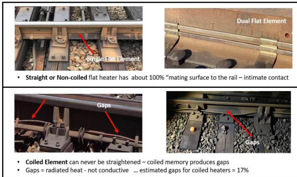
Figure 9 Comparison of Installations between Straight Element (top) and Coiled Element (bottom)
